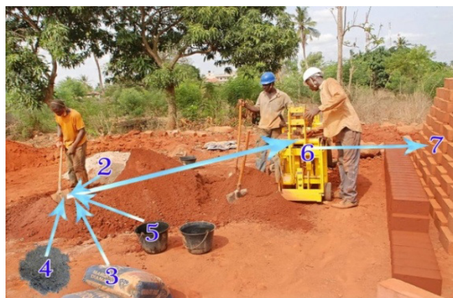
Figure-3: dosage and mixing dry red soil to cement and wood sawdust K. senegalensis .
