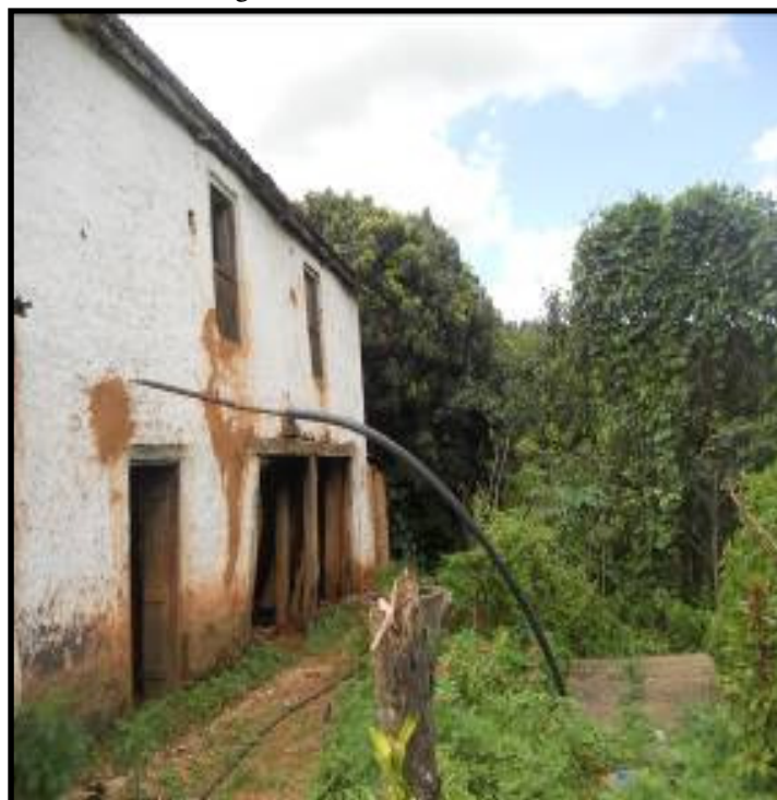
Figure-2 A A pipe connecting kitchen sink (inside)
