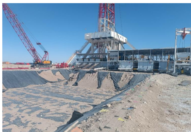
Figure-2: Drilling rig and wastewater storage.
