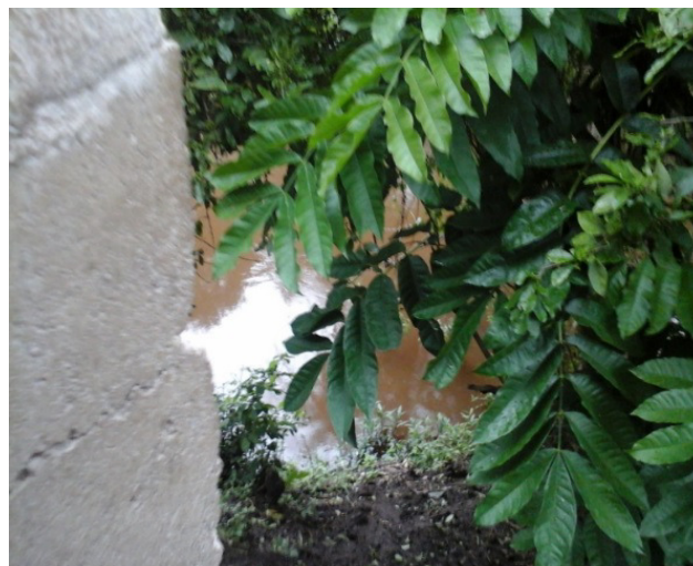
Figure-7: Wall of a building raised next to the river waters.
