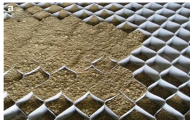
Figure-1 A typical geocell 15
