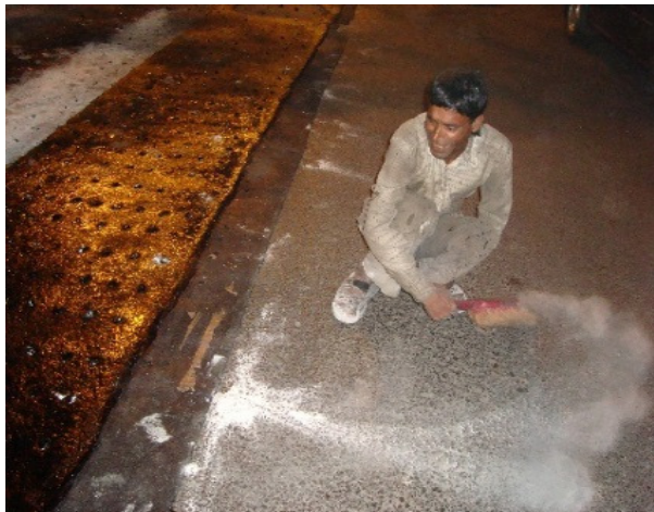
Figure-6 Cleaning of road surface
