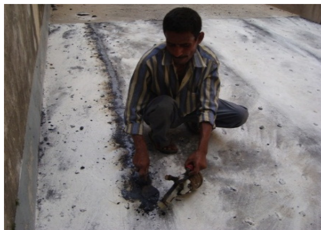
Figure 11 Thermo sealing of the joints
