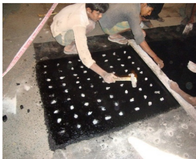
Figure 10 Placing of antiskid stone chips
