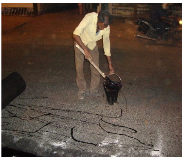
Figure-7 Application of tack coat
