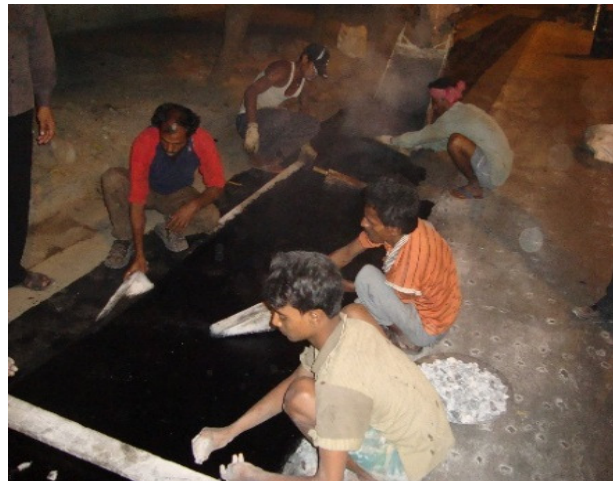
Figure9 Laying of mastic on BJPF
