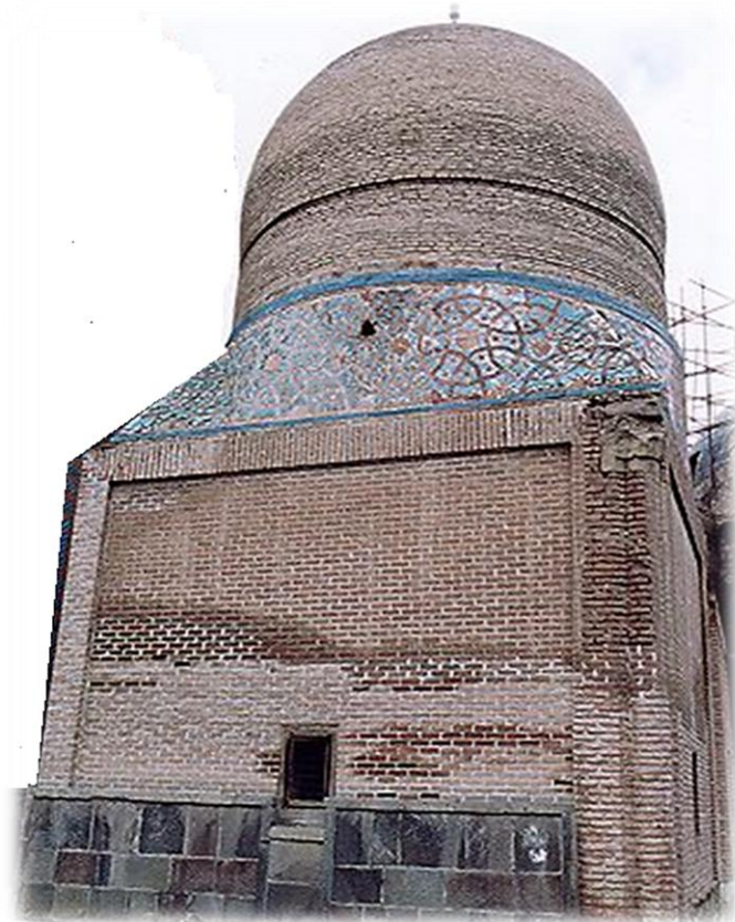
Figure-9 Dome of building Haram-khana
