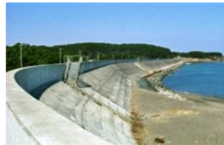
Figure-3 Massive concrete wall along the coast
