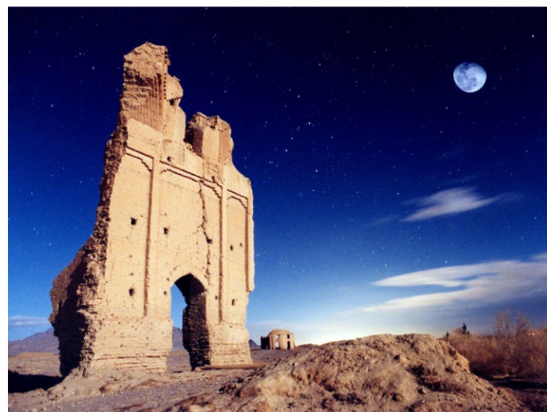
Figure-3 Surviving gates of the Safavid era
