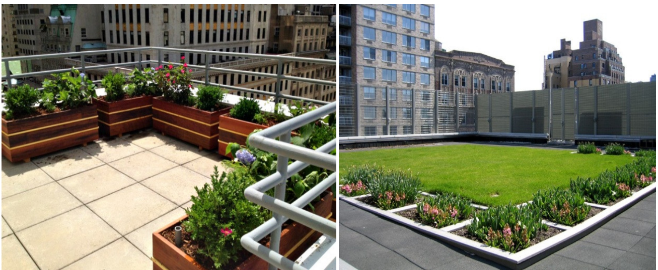
Figure-1 An instance of using plants of the roof
