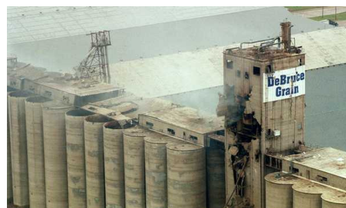
Figure-0 After explosion in DeBruce Grain Company 13
