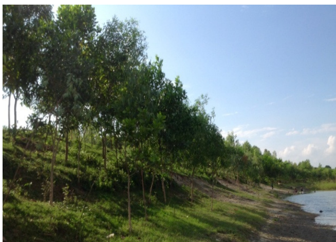
Figure-4 Riverside Forestry on embankment
