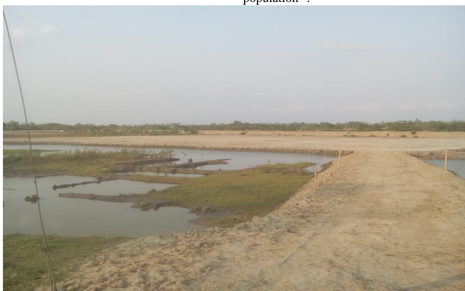
Figure-6: Tidal creek closure project.
