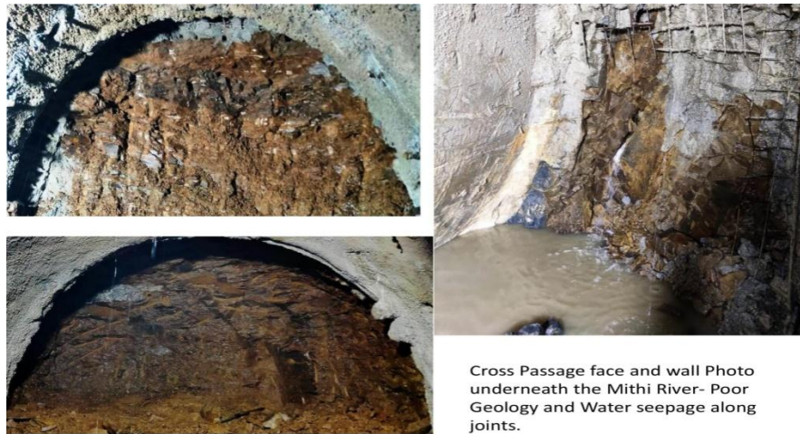
Figure-13: Rock face and water seepage during construction of cross-passage underneath the Mithi river.
