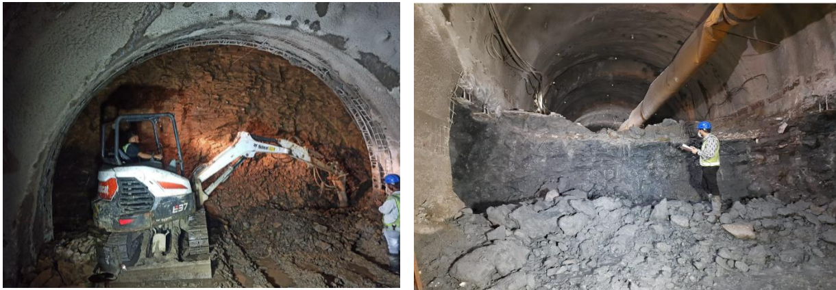
Figure-12: Heading and benching excavation under BKC south NATM tunnel.
