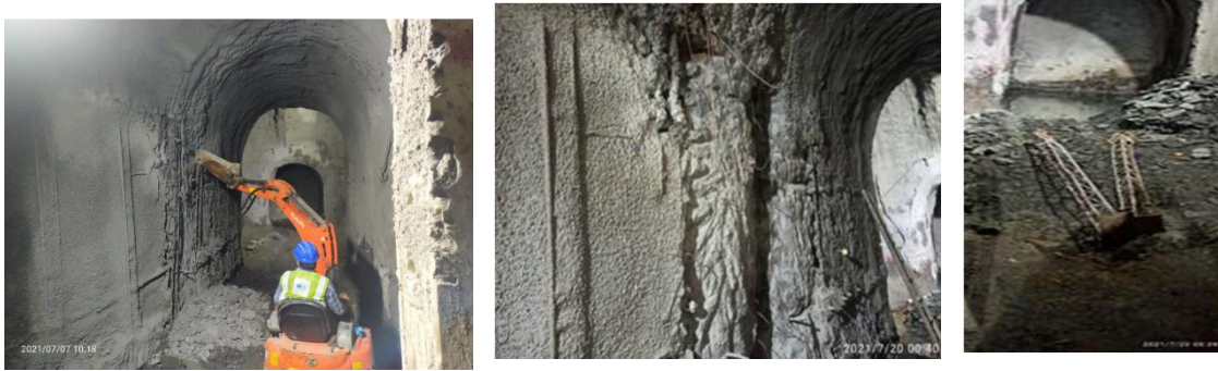
Figure-14: Repair of undercutting work.
