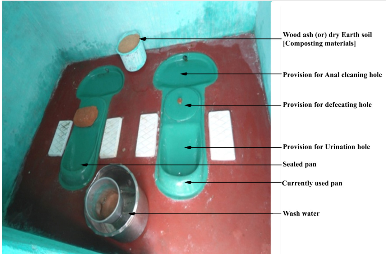
Figure-2: Inside view of Eco-san Toilet.
