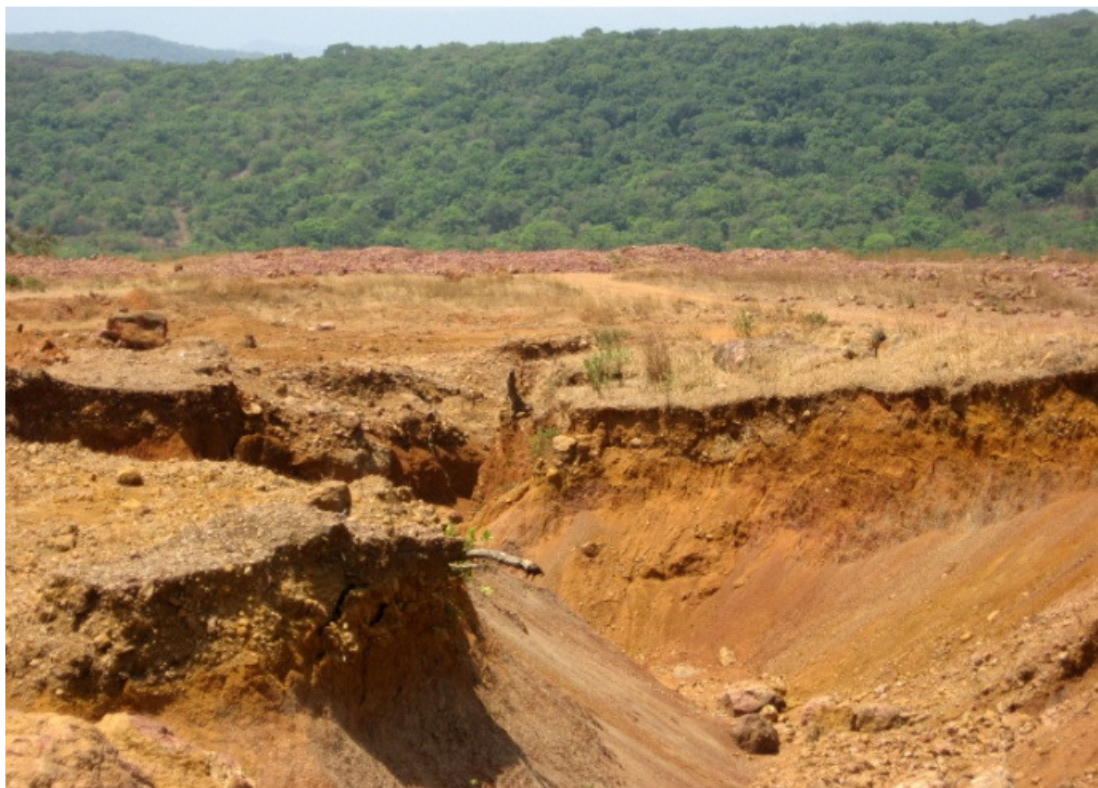
Figure-2 Diversion of natural stream at bauxite mine M/S Prakash Anandrao Gaikwad
