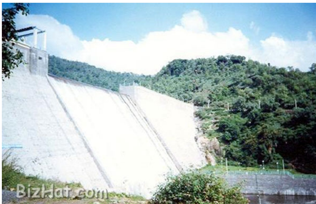
Figure-2 Sothuparai Dam
