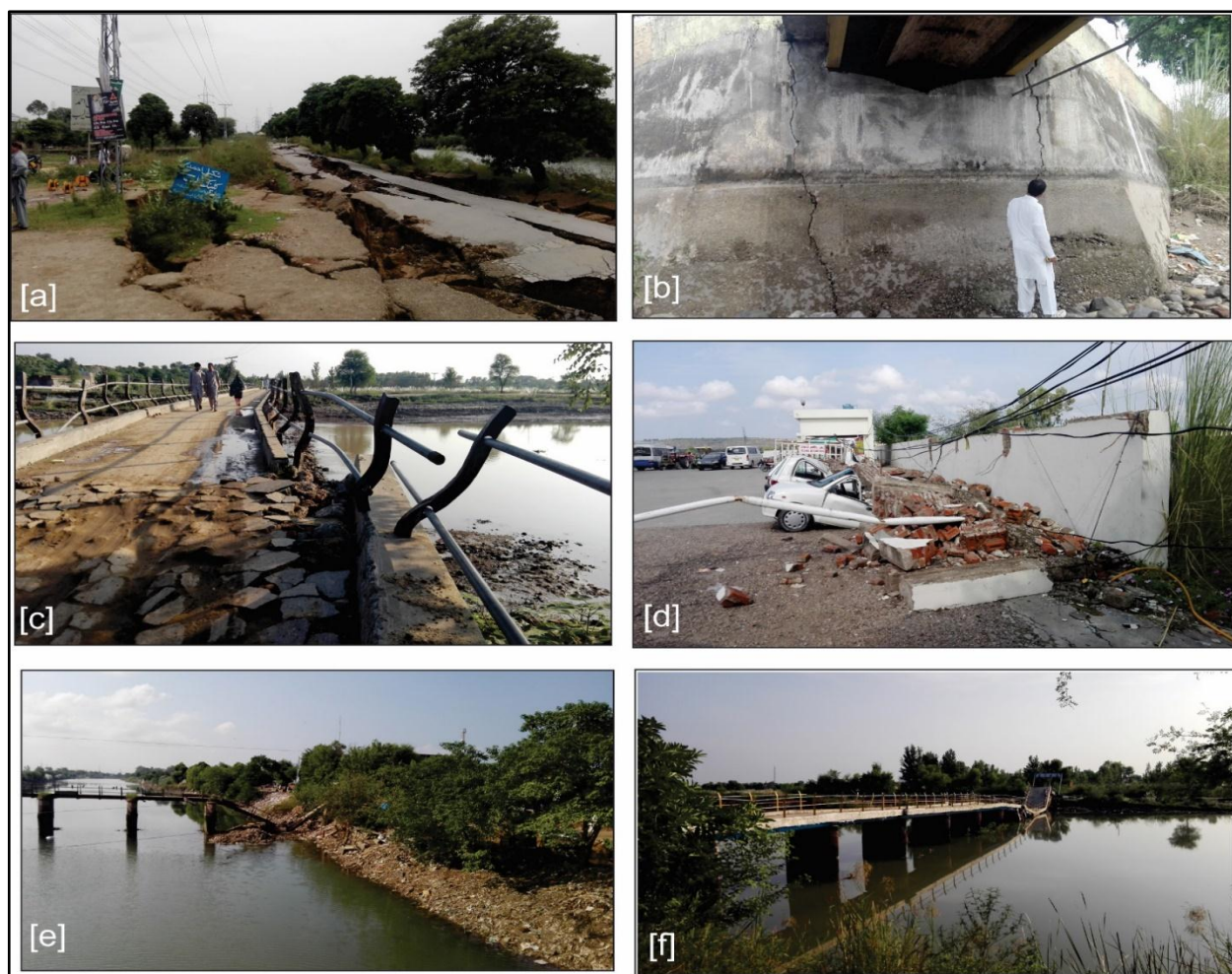
Figure-10: Field photographs showing (a) the liquefaction induced lateral spreading along the embankment of UJC (b) cracks in abutment of Dab Bridge (c) vehicle damaged by the collapse of boundary wall (g) Manda Bridge collapse (e) the Bani Bridge after earthquake (f) the displacement of abutment of Sang Bridge.
